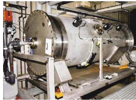
RBR heterotropher Nitratfilter
