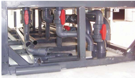
last works inside the tank tubing made of PVC
