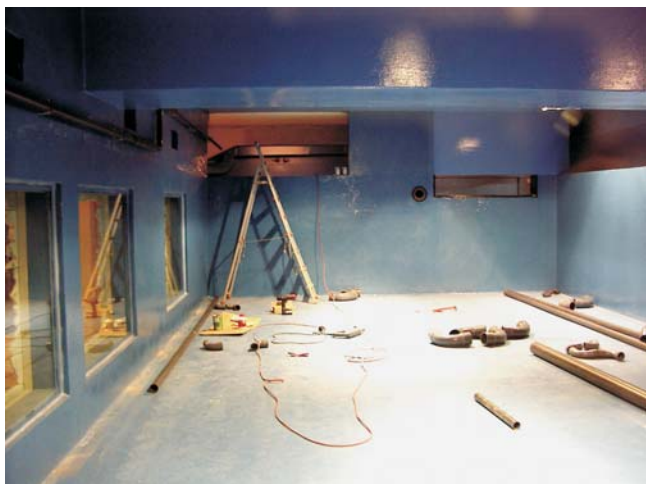
inside of the tank in construction
