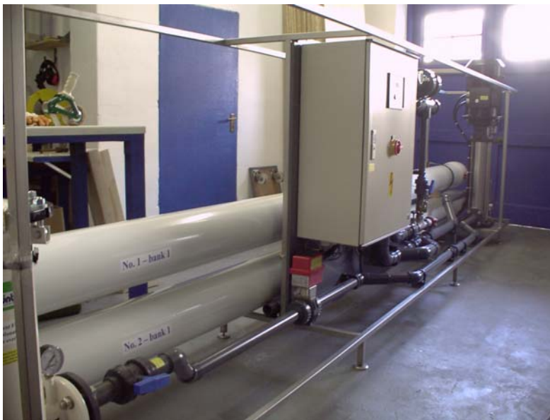
Stainless steel tubing with VICTAULIC connectors
