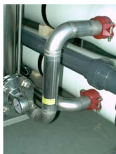
Stainless steel tubing with VICTAULIC connectors
