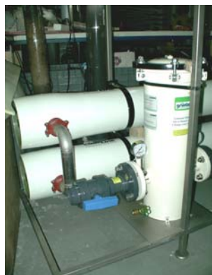
sediment filter made of stainless steel covered with plastic
