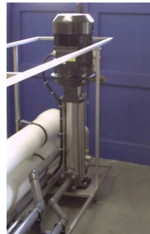
Multi stage high pressure pump made of stainless steel
