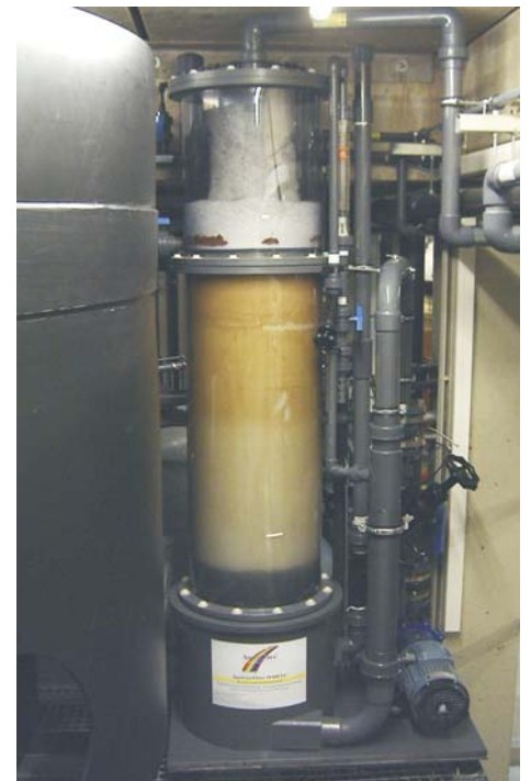
modified skimmer to eliminate bacteria and traces of nitrite
